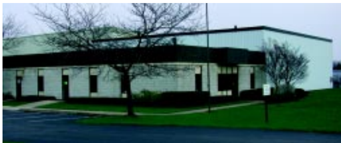
Above, the exterior of Winkle Electric's new distribution center and sales office in Erie.
